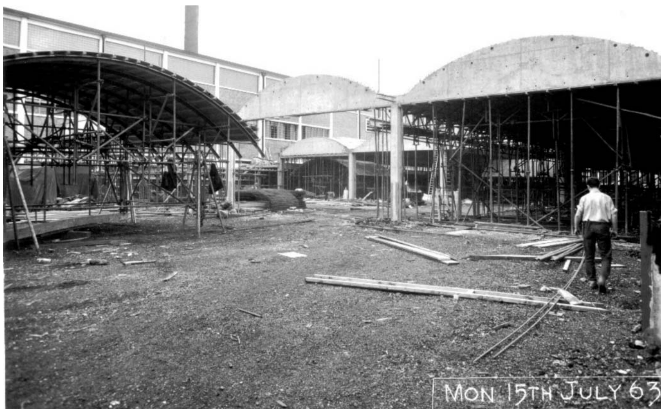
Figure 10. New Salle, Building 25: under construction, 1963 ( Apsley Paper Trail )
